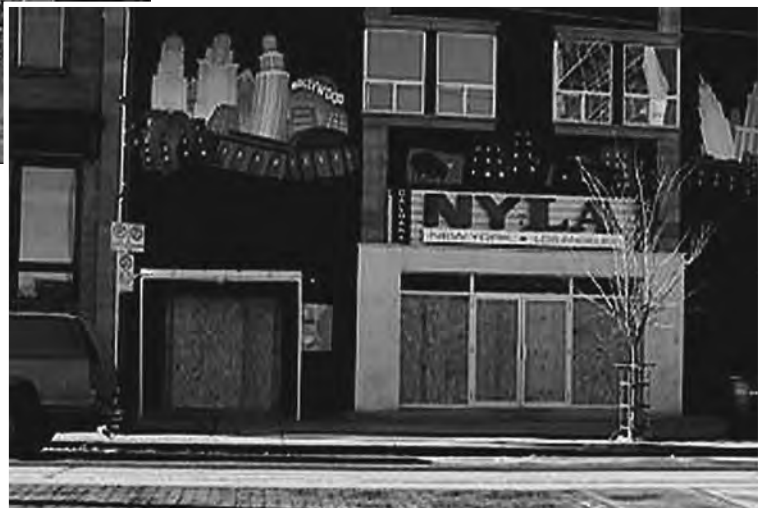
Figure 4 Boarded up exterior windows, 2003
