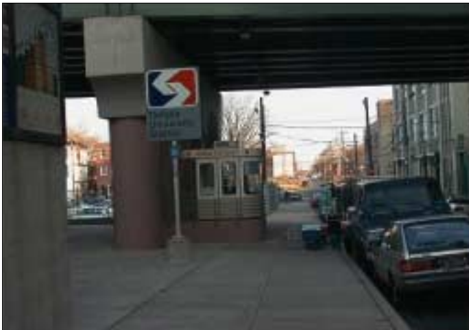
Figure 1. Train Station Security Kiosk
