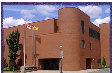
Police Station, 311 Queen Street
