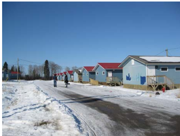
Picture 5. The current school delivered through a system of portables. Note graffiti on the walls of the buildings March 5, 2010.
