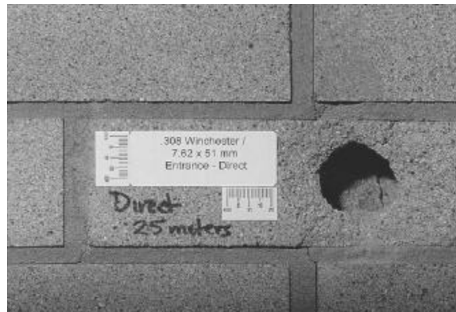
Figure 3 - Damage to clay brick caused by .308 Winchester
