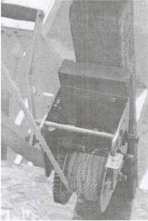
Photo 1. Winch connected to main rope.
